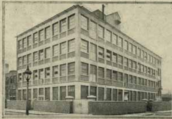
A View of the Matchless Works. Especially noticeable is the large window area, giving ample interior light.
