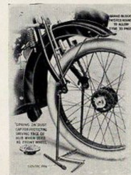
Showing Front Wheel detached and its interchangeability with Rear Wheel
